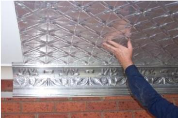
4. This picture shows the sheeting then going over the top edge and butting up ready for fixing in place. Sheeting can be started from the centre of the room or the cornice edge.
