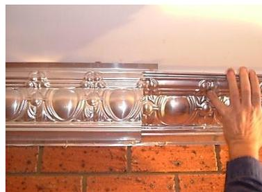
7. Install the next length of cornice into the mounting strip, overlapping the previous cornice. Some paintable no-more gaps may be smoothed over the joint to help it to appear seamless.
