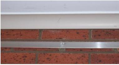
1. Begin with the Cornice Mounting strip. This needs to be glued and fixed into place along a level line, marked at the correct height for your cornice. Lip is to face out.
