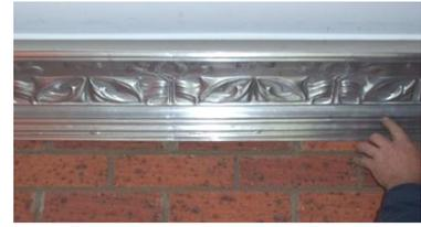
3. Shows the Cornice in place, which you can install straight over an existing Gyprock Cornice. Then affix the top flat cornice edge into your ceiling with nails, tacks etc
