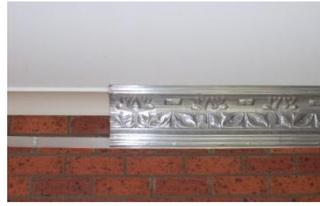
2. This picture shows the cornice slipping into the Mounting Strip.
