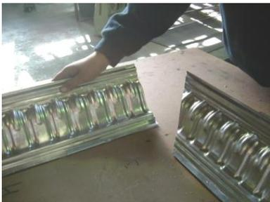
4. Picture shows left hand Cornice piece remains "square", to be installed as is. Right hand cornice has been mitred and scribed to fit profile of left hand piece.
