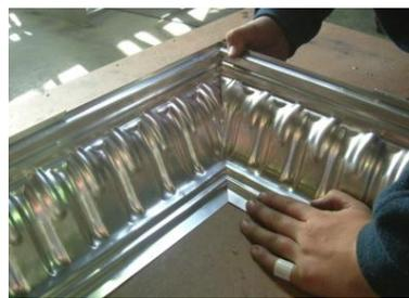
5. Picture shows both cornices coming together, just as they will be when installed. Minor trimming may be required to perfect the joint.
